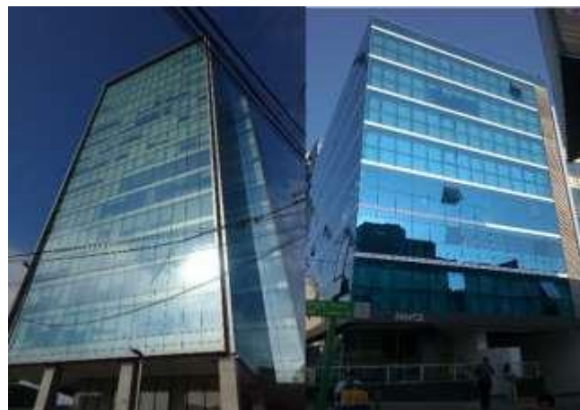
Figure 2. Leuro and Cantuarias Buildings in Miraflores
